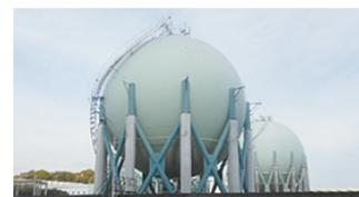
Brace retrofitting on a spherical tank
