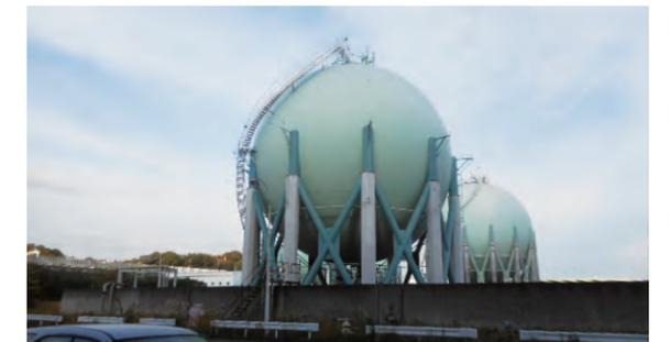
Brace retrofitting on a spherical tank
