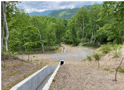
Stone tailings drainage at Toyoha Mine
