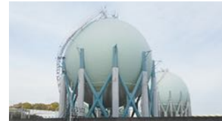
Brace retrofitting on a spherical tank
