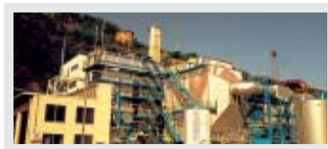
The rotary incinerator at Nikko Environmental Services Co.,Ltd. (Ibaraki prefecture)
