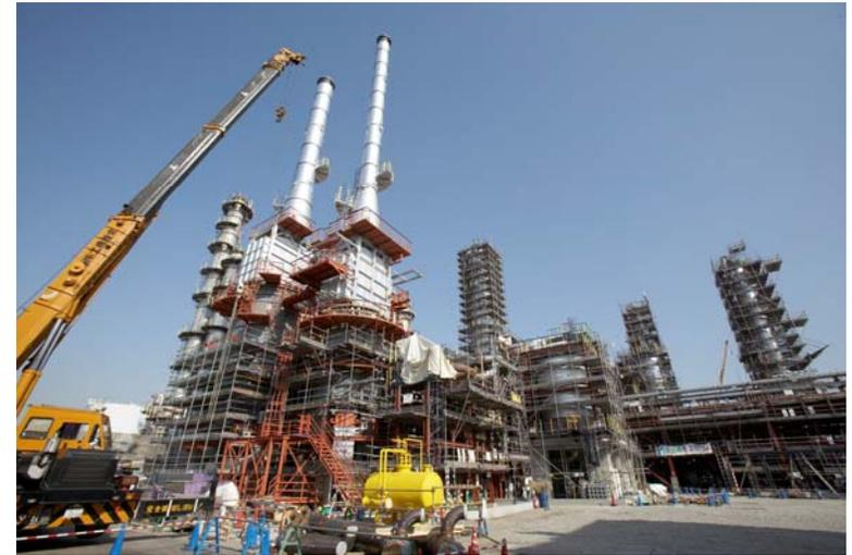
New unit to produce low sulfur petroleum products at Kawasaki Refinery
