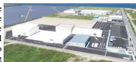
Oita Recycling Logistics Center
