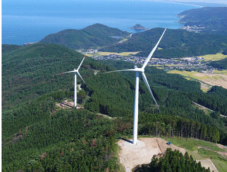
Tsuruoka Hachimoriyama Wind Farm, Japan Renewable Energy Corporation
