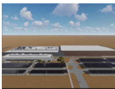
Completed new overseas plant as imagined
