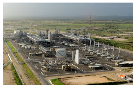
Facilities of the PNG LNG Project (Papua New Guinea)
