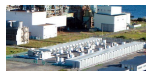
Muroran storage battery system
