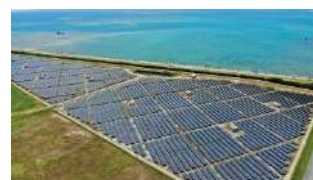
Uruma Mega Solar Power Plant
