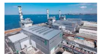
Goi Thermal Power Plant
