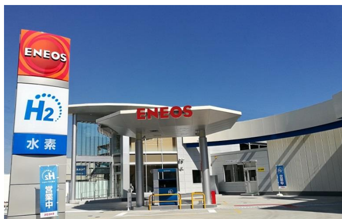
Hydrogen station (Kohoku-ku, Yokohama City)
