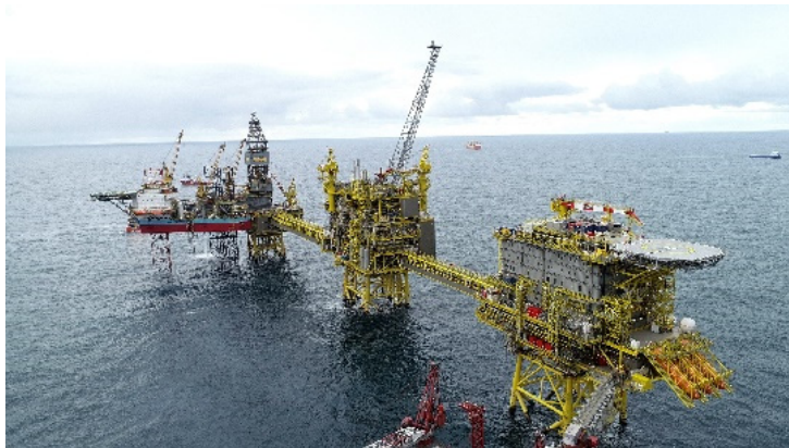
Culzean Gas Field Offshore Facility (UK)
