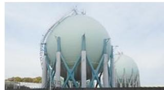
Brace retrofitting on a spherical tank
