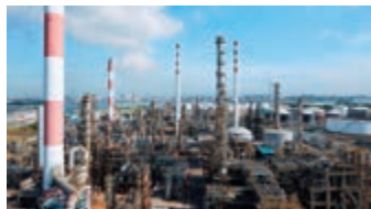
Singapore Refining Company
