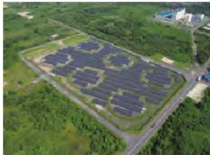
Kudamatsu Mega Solar Power Plant
