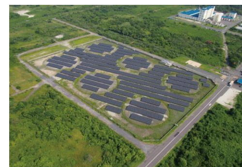
Kudamatsu Mega Solar Power Plant
