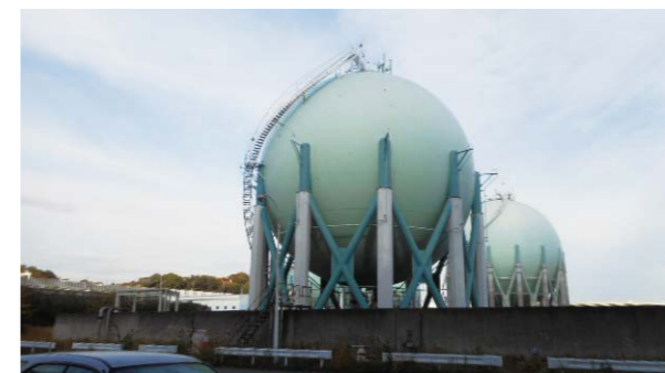
Brace retrofitting on a spherical tank
