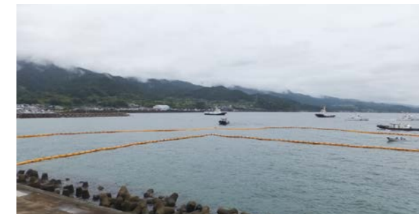
Deploying an oil fence during a drill for a marine oil spill
