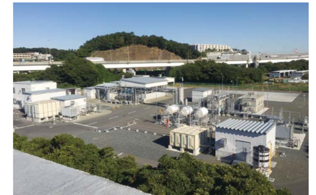
Hydrogen Manufacturing and Shipment Center (Naka Ward, Yokohama City)
