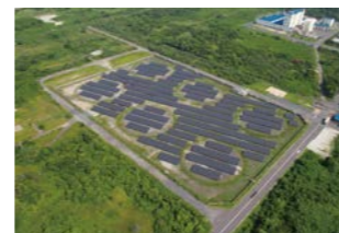
Kudamatsu Mega Solar Power Plant
