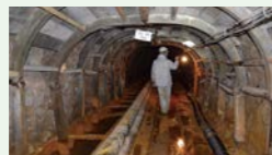
Gallery inspection at Hanawa Mine
