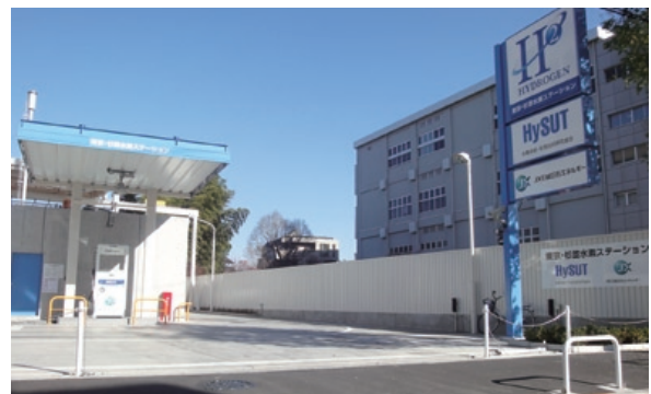
Tokyo Suginami Hydrogen Station
