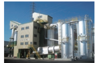
NIPPO CORPORATION's Kyoto Asphalt Mixture Plant, which recycles asphalt pavement
