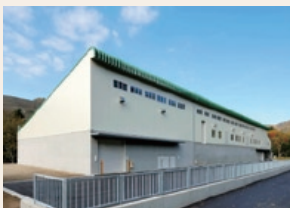
Exterior view of the wastewater treatment facility
