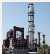
Atmospheric distillation unit at the Mizushima Refinery
