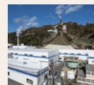
Hitachi Metal Recycling Complex (HMC) Works
