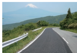
The Ashinoko Skyline toll road, operated by Ashinoko Skyline Corporation, which is 100% owned by NIPPO CORPORATION.
