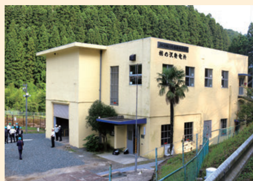
The upgraded Kakinosawa Power Plant
