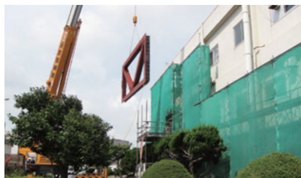
Seismic reinforcement of buildings
