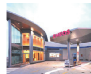
Yokohama Tsunashima Hydrogen Station and Suiso Terrace
