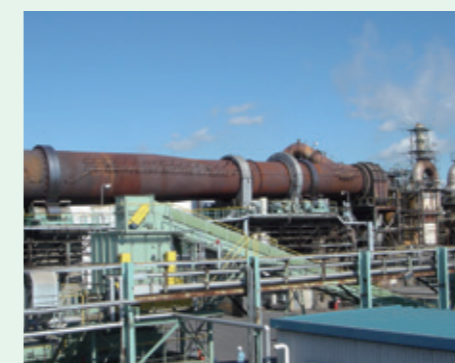
JX Nippon Tomakomai Chemical rotary kiln furnace
