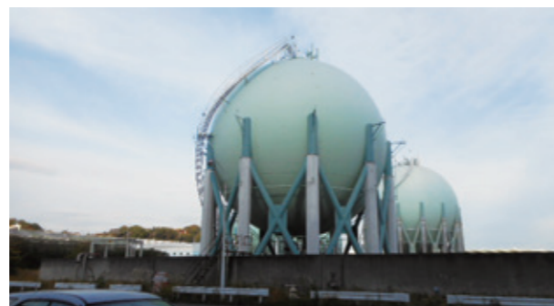
Brace retrofitting on a spherical tank
