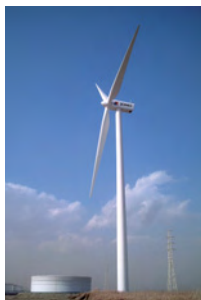
Wind power generation facilities at the Kashima Oil Refinery
