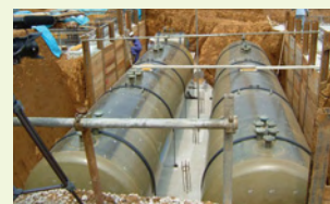
Renewal work for double-walled tanks
