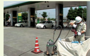
Soil contamination investigation
