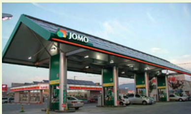
A JOMO service station installed with solar panels for power generation
