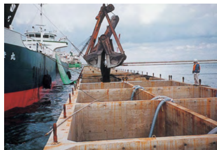
Filling caissons* with copper slag
