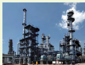
Paraxylene production facility at the Chita Oil Refinery
