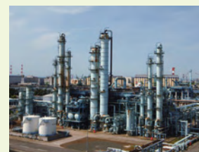
Aromatics production facility at the Kashima Oil Refinery
