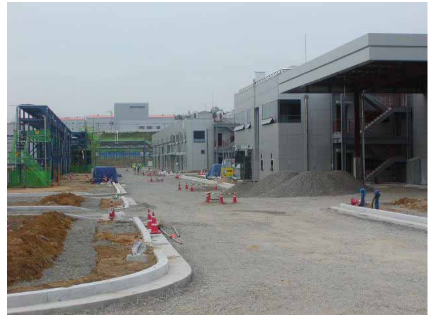
New BSF Production Facility Construction (Gumi City in Korea)
