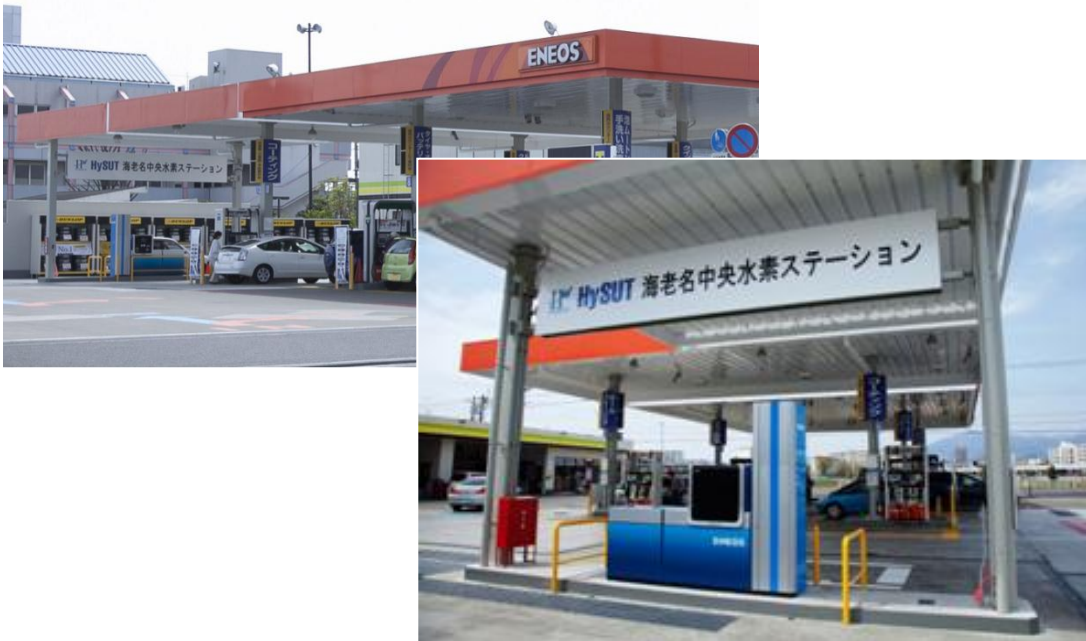
Service Station (SS) that has Gasoline and Hydrogen Filling Machine (in Kanagawa)
