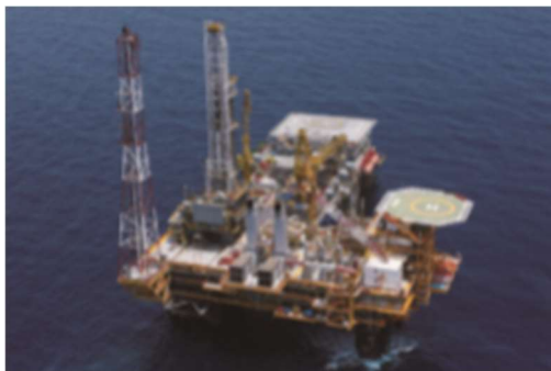
Helang Gas Field Offshore Facility (Malaysia)
