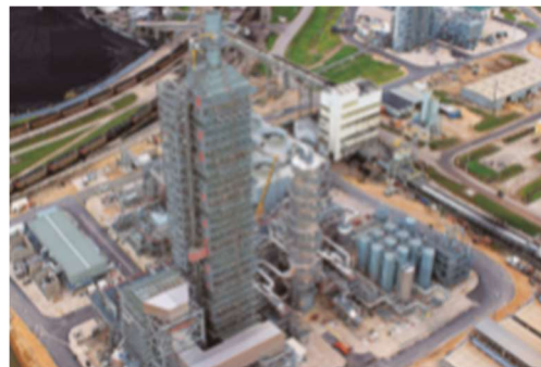
CO2-EOR Project in the U.S. CO2 Recovery Plant
